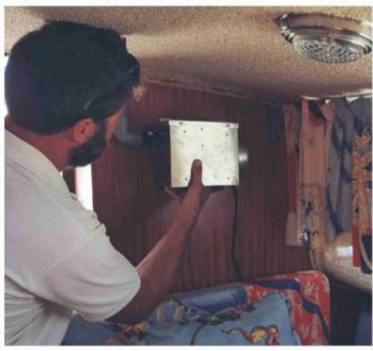
panel, far right) was fairly straightforward: go desiccant. Desiccant dehumidifiers work better than compressors in cooler air temperatures and they produce clean, dry air that is a good 10°C warmer post drying – fulfilling two roles at once.
